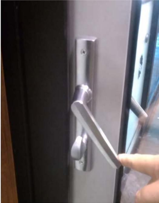
To open the door, after unlocking, push handle down and push door out.
