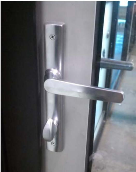
This is the handle on the swing door and is shown in neutral and or locked position. If the door is locked turn the thumb-turn (lower part) and you will feel and hear the dead latch, unlock. In this case it would be an anti-clockwise turn. Opposite door will turn opposite.
