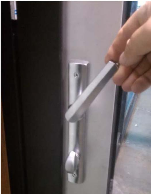
To close the door tightly against the weather, pull the handle lightly toward you and turn handle up, as shown. You will feel and hear the dead bolts and shoot bolts engage.
